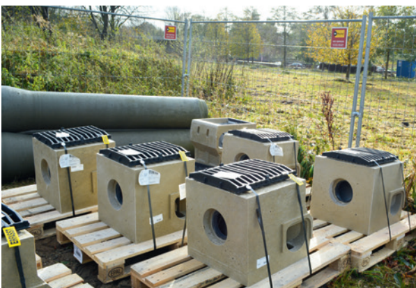
Baffle wall shafts ready to install
