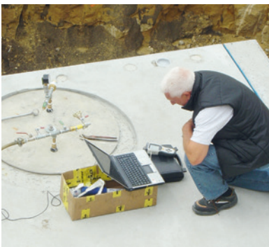
Use compressed air to check tightness
