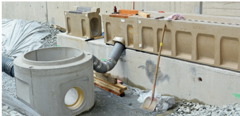
Connecting element with siphon pipe to the control shaft and connection to the longitudinal drainage guide
