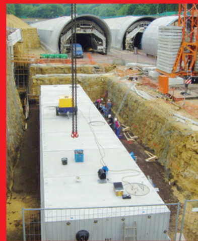
ACO large containers as emergency tanks
