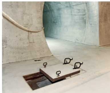
Open shaft manhole cover
